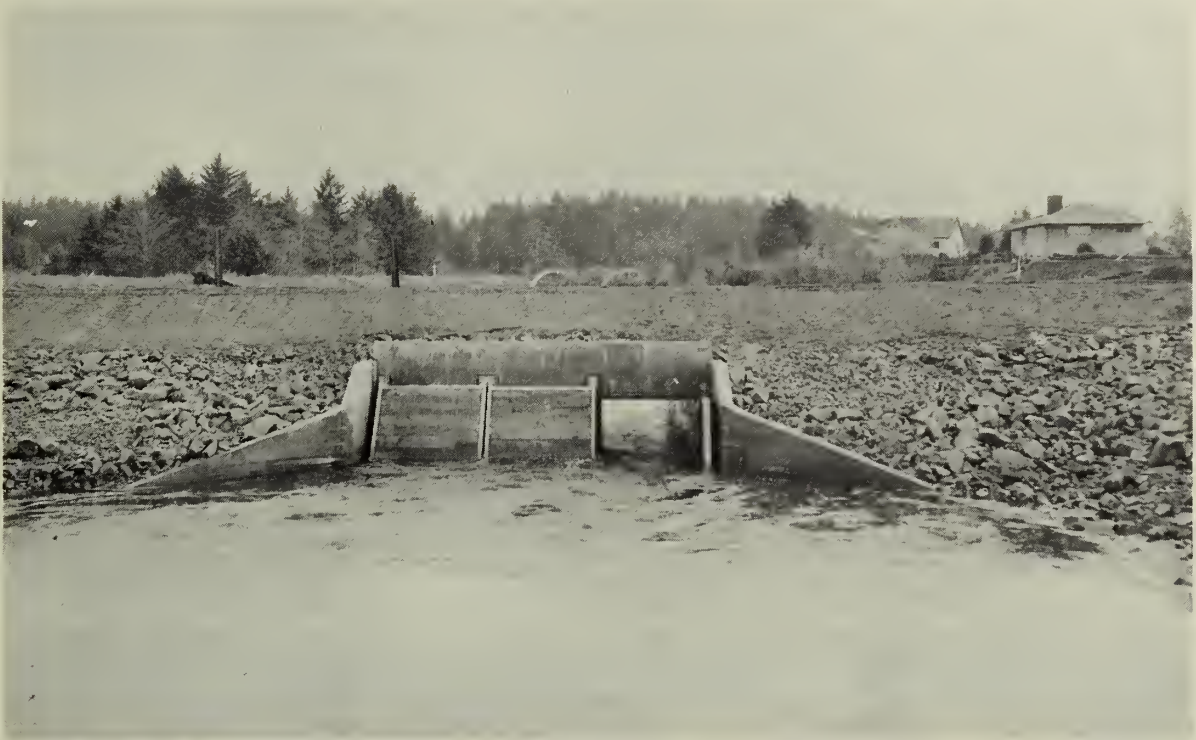
Photo 38.--These flood gates on the Skipanon River are part of the P. L. 566 project near Warrenton. SCS photo
